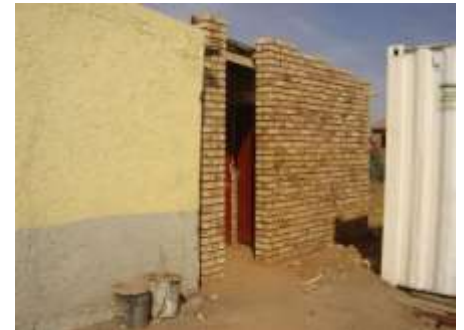
Work in progress as at 28 July 2011.
